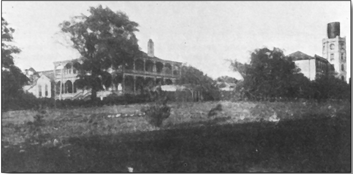
Superintendent's Office at Chattahoochee, residence and water tower, circa 1905.
