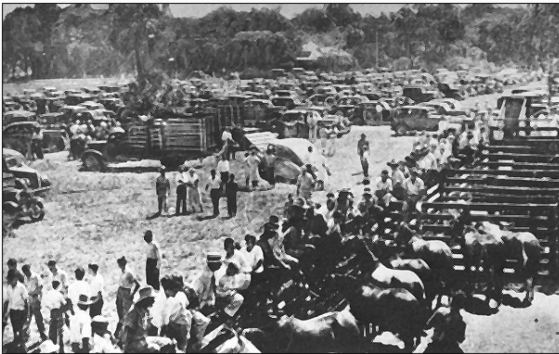
The WPA also built this livestock market in LaBelle.
